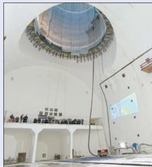
On 1 February 2005, the cavern for the CMS detector at CERN was inaugurated in a ceremony attended by many guests, including representatives of the construction companies.
