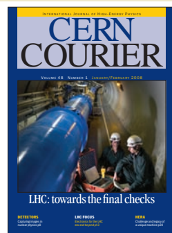
The LHC is on course to start up in 2008, with the machine components fully installed and commissioning well underway.
