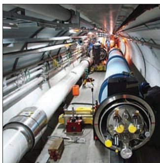
On 5 September 2006 the 1000th superconducting magnet system was installed in sector 3-4. During the same week, the final system for sector 8-1 was also installed.
