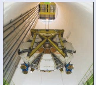
The final large piece of the ATLAS detector was lowered into the underground cavern on 29 February 2008. The “small” muon wheel safely made the 100 m journey in an hour and a half. ● April 2008 p5.
