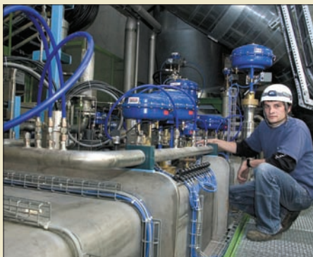
The cryogenic unit at Point 8 has reached its nominal temperature of 1.8 K.
