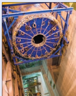
In January 2007 the fragile 5 m diameter time projection chamber (TPC) weighing 8 tonnes was lowered into the cavern. (Courtesy A Saba for CERN.) ● March 2007 p6.
