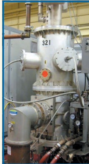
5 MW Cavity Amplifier
