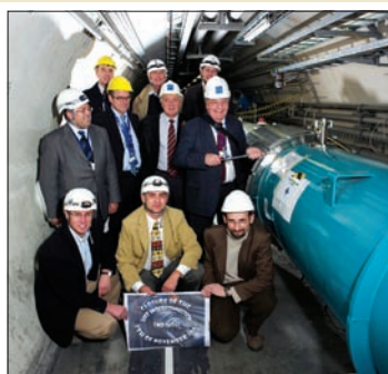
Director-general Robert Aymar sealed the last interconnect between the main magnets on 7 November 2007, at the end of two years of work involving 123 000 connections.
