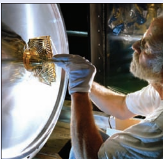
The first beryllium section of LHCb’s beam vacuum chamber was installed at the end of August 2006. Here, a technician inserts the wakefield suppressor.
